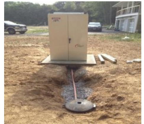
Hydrogen Tank Connected
